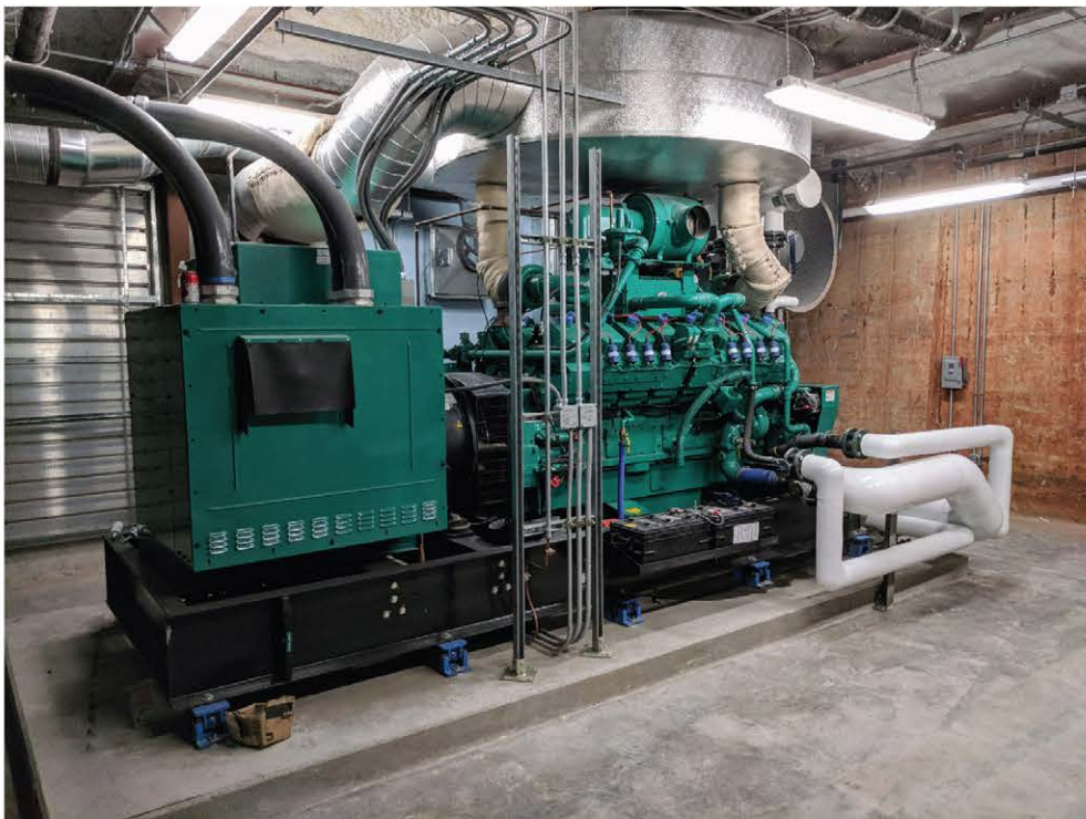
Top: A crane carefully lowers the Capitol's new emergency power generator into place. Bottom: The completed emergency power generator weighs over 24,000 pounds and generates 828 kilowatts of electricity.
