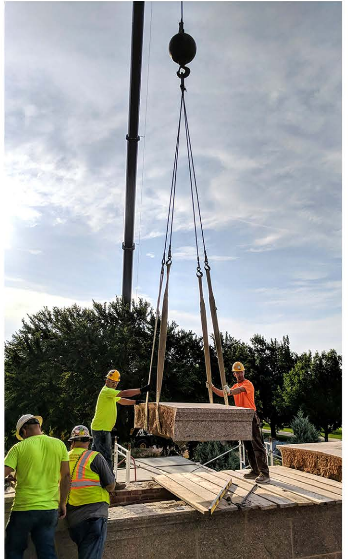
Top left: Workers pour concrete on a new structural support system for the Capitol's north stairway. Bottom left: Engineers discovered many of the Capitol's exterior stairways were structurally unsound. Right: Stonemasons reinstall large granite blocks weighing several tons on the south side of the Capitol.
