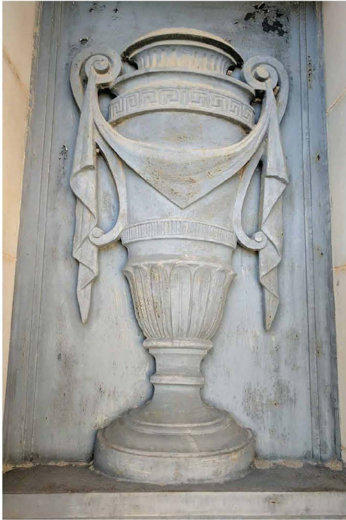
This decorative cast iron urn on the south wing of the Capitol was in poor shape prior to its restoration.
