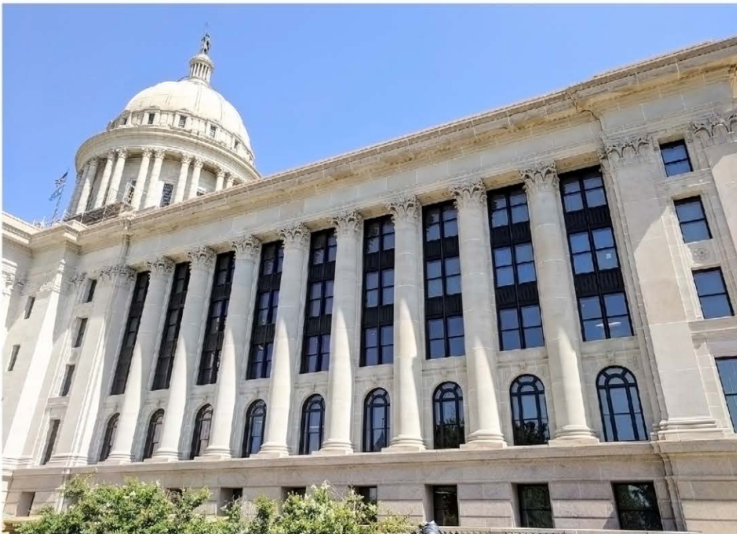
Top: Scaffolding is removed from a completed elevation on the east wing of the Capitol. Bottom: A completed elevation of the building includes restored windows, repaired limestone, newly cleaned limestone, new gutters, and new mortar in the stone joints.
